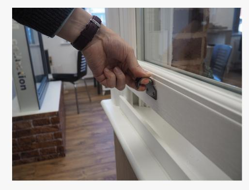
Unlock the cam catch(es) with the key supplied, and turn the lever(s) anticlockwise to open.
