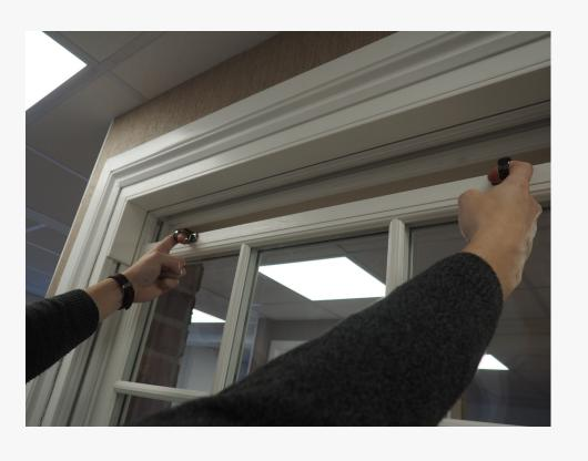
To open the bottom sash, raise the sash using the lift handles.
