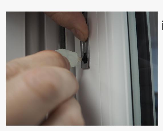
With one hand push and hold the limit stop in, and then with the other hand turn the key.
