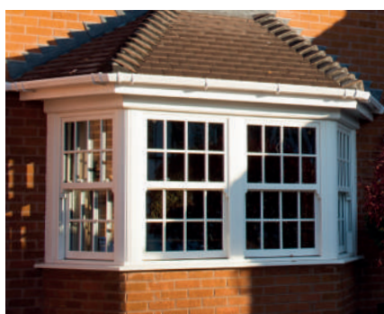
Bay window with vertical sliding sash windows
